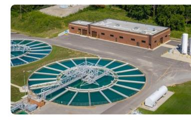
The facility was upgraded with ozone in 2020 to improve water quality and allow WaterOne to proactively meet future drinking water regulations. In addition, ozone allowed WaterOne to operate more efficiently and cost effectively and is projected to pay for itself within 20 years due to reduced operating expenses.
